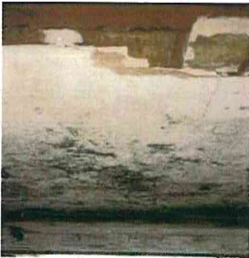
Photograph No. 5 View of rough textured drywall located on walls.
