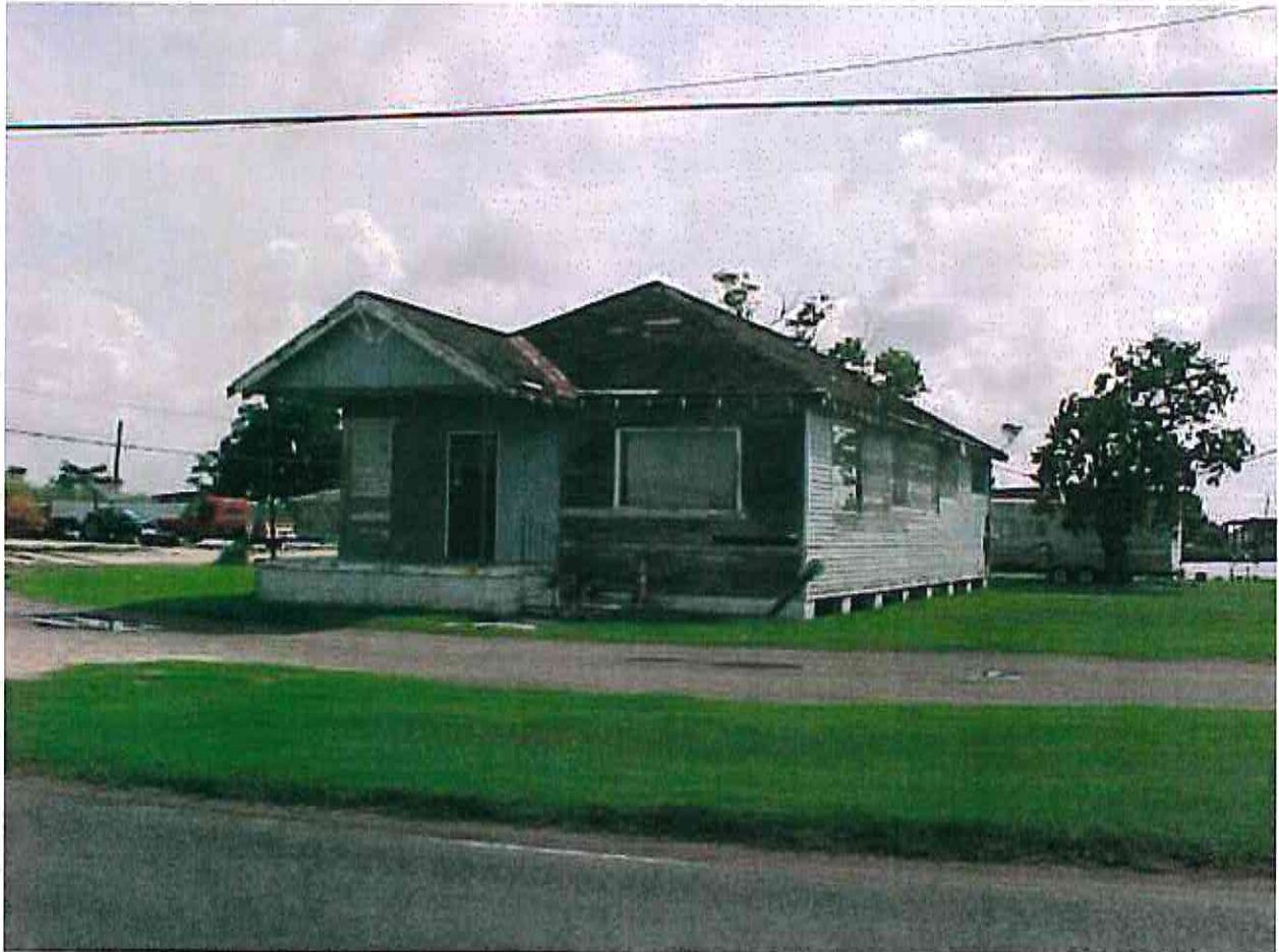
A SIGN IS POSTED ON THE BUILDING TO BE DEMOLISHED
