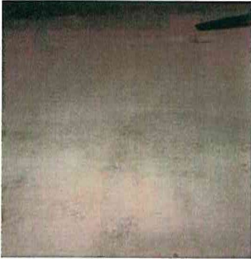
Photograph No. 6 View of smooth textured drywall located on walls.
